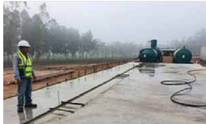
CCA treatment plant when nearing completion of civils
