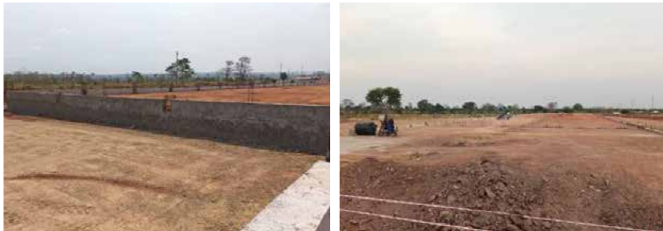
Plymill construction (foundation completion stage)
